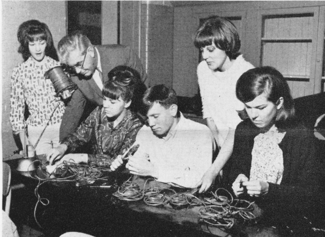
SOLDER ASSEMBLY. Measuring and cutting proper lengths of wire, preparing one end for plug attachment and the other for insertion into case assembly are Kathie Grant, Grazina Melninkas, Dave Newell, Vida Lipkis and Debbie Stokes, under the watchful eye of Adviser Bob Pierson.
